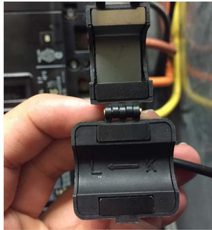
Use the required amperage CT clips and install to the desired circuit(s) that you want to measure.
